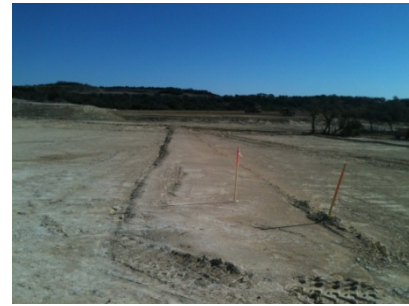
6 PARKING LOT GRADING
