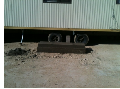
3 FOUNDATION FOR MOCK WALL
