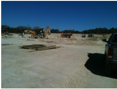
4 PLUMBING WORK AT AREA A
