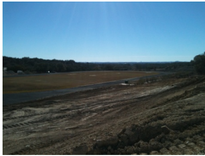
5 VIEW TO SE OF TRACK
